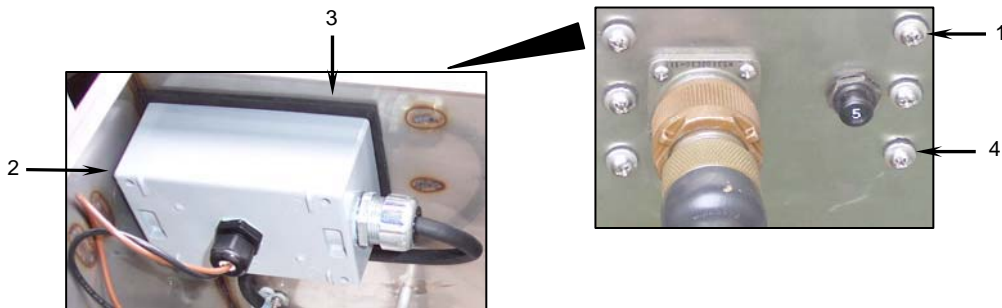
Figure 5. Installing the Grease Separator Weatherproof Box.
