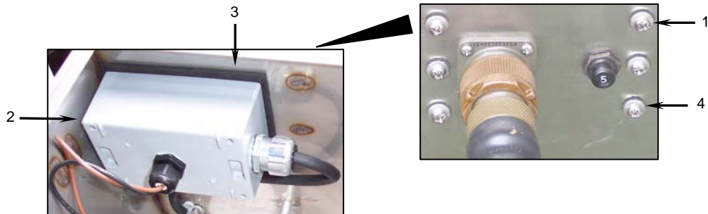
Figure 6. Installing the Grease Separator Weatherproof Box.
