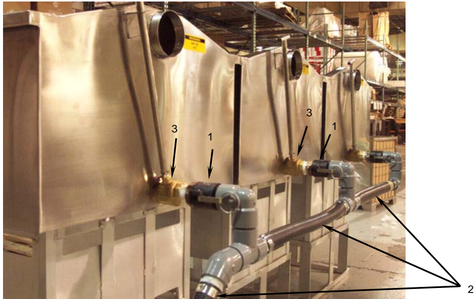
Figure 14. Sink Drain Hose Assembly Installation.
