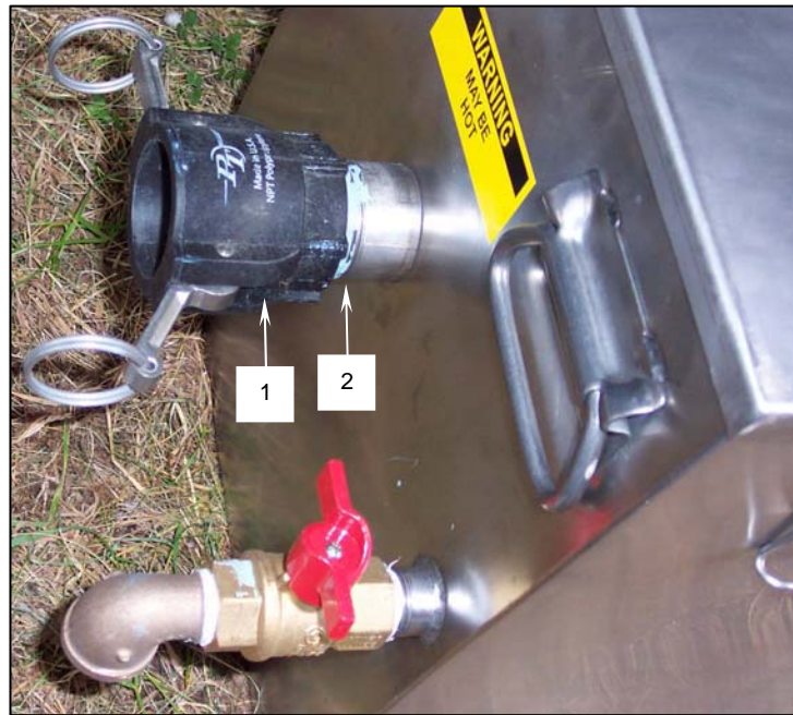
Figure 1. Replacing the Grease Separator Inlet Coupler.
