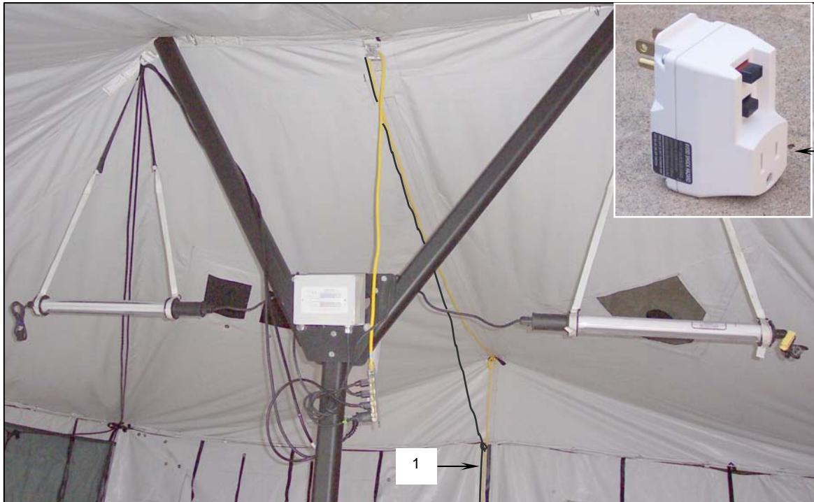
Figure 33. Unplug 100-ft Extension Cord and GFCI.
